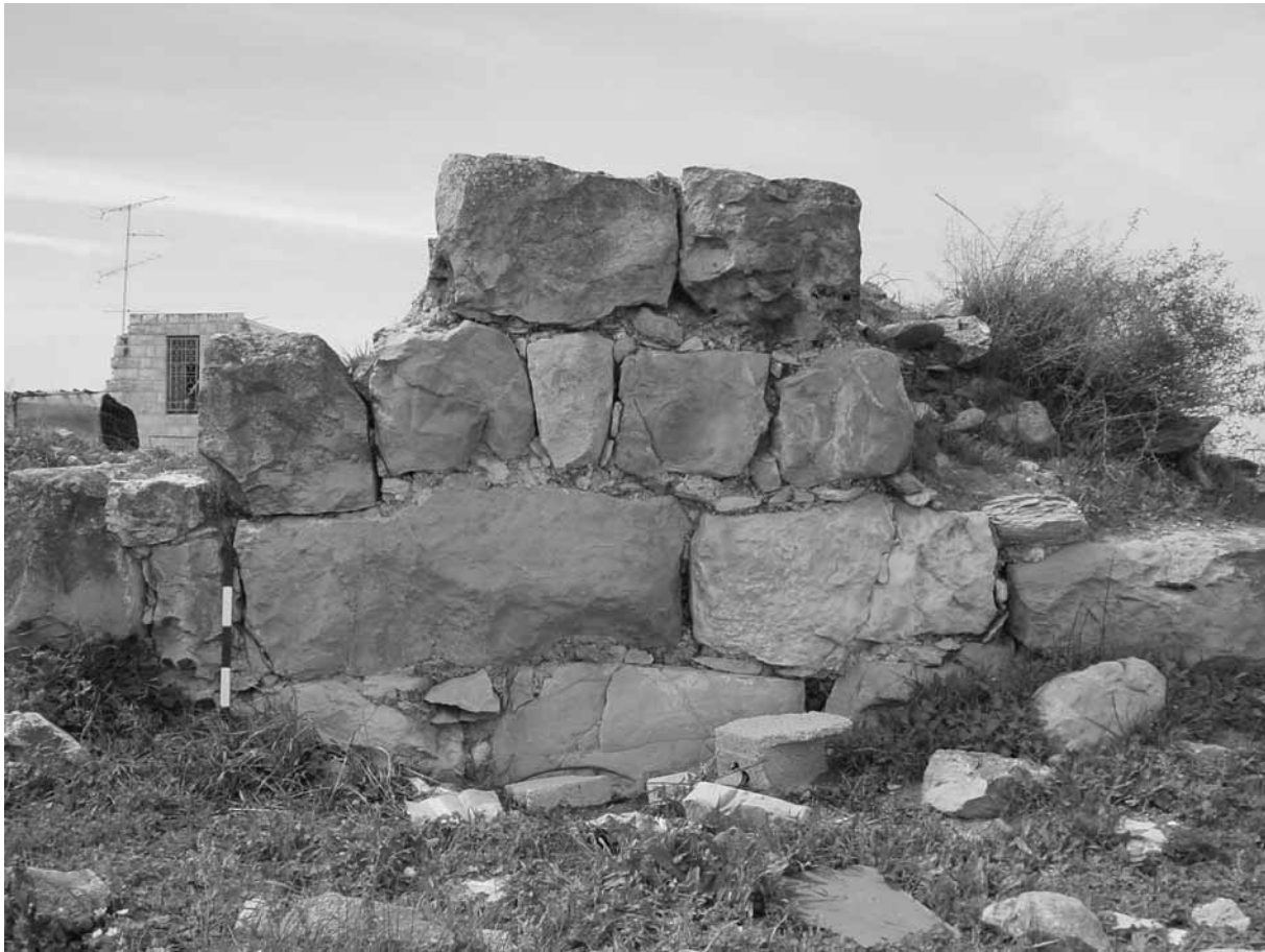
Figure 15. East wall of the tower-like structure on the summit of Khirbet es-Sauma'a. Photograph: S. Gibson.
